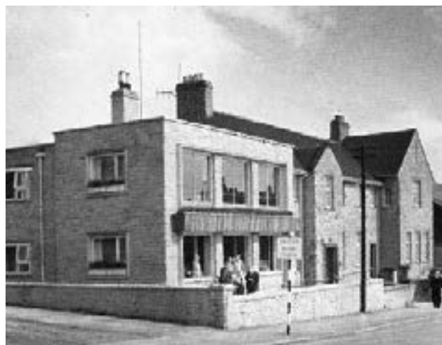
Completed extensions at Cairn Home
